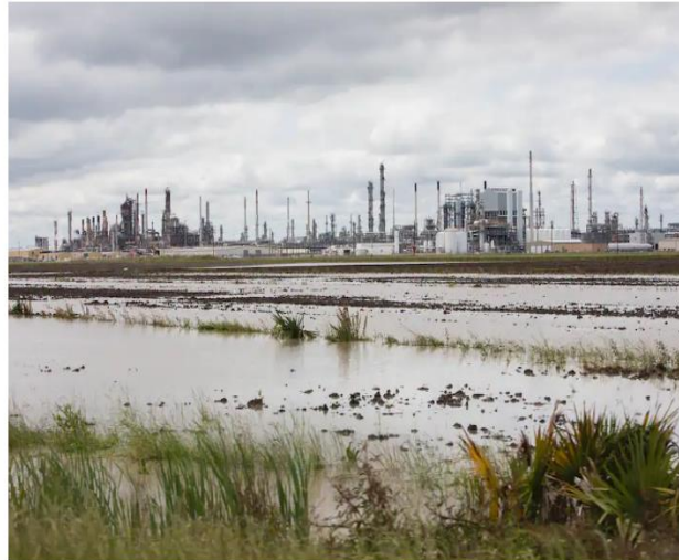
Industrial plants and flooded farmland cover much of the landscape in St. James Parish, La., not far from where Formosa hopes to build a huge plastics manufacturing complex. (Camille Lennain for The Washington Post)
